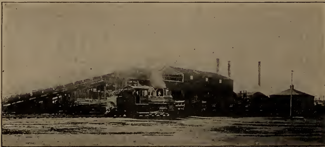
COLLIERIES AT WESTVILLE, NOVA SCOTIA.
